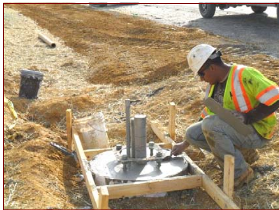
Job No.: 07-14-00, A Joint Venture of Shirley Contracting Company, Facchina Construction Company, Clark Construction and Trumbull Corporation @ ICC, Contract C: Jose Guidel and Dery Guidel finishing concrete for light pole foundations.
