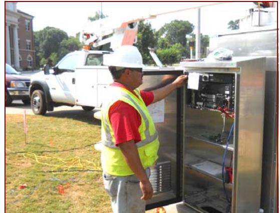
Job No.: 10-18-00, Coweta County, GA @ Traffic Signal Upgrade: foreman Baldemar Avalos installing a back up battery cabinet.
