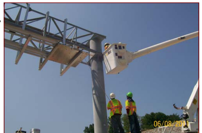
Job No.: 06-16-00, Fluor/Lane, LLC @ I-495 HOT Lanes: Installing cantilever sign structure.
