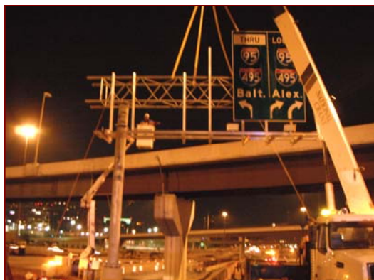
Job No.: 07-15-00, Corman and Kiewit Joint Venture @ Telegraph Road Interchange: Helmer Andrade and crew members installing a cantilever sign structure.
