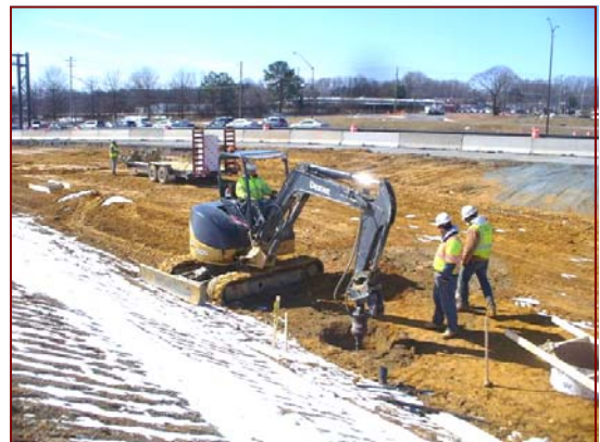
Job No.: 07-14-00, A Joint Venture of Shirley Contracting Company, Facchina Construction Company, Clark Construction and Trumbull Corporation @ ICC, Contract C: foreman Henry Guidel and crew digging light pole foundations.
