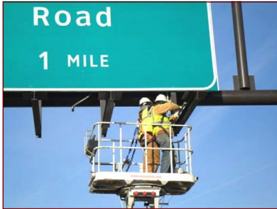
Job No.: 07-14-00, A Joint Venture of Shirley Contracting Company, Facchina Construction Company, Clark Construction and Trumbull Corporation @ ICC, Contract C: Foreman, Johnny Herring and crew installing electric conduit on a sign structure.
