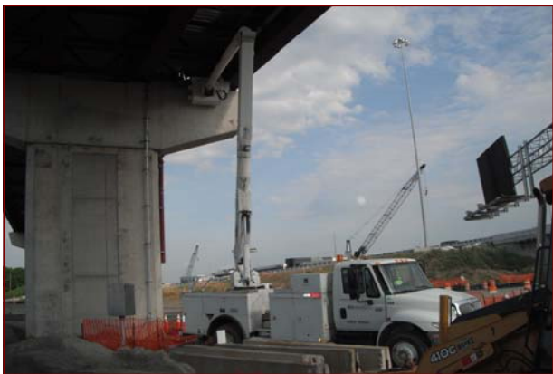
Job No.: 07-15-00, Corman/Kiewit Joint Venture @ Telegraph Road Interchange: Crews pulling fiber.
