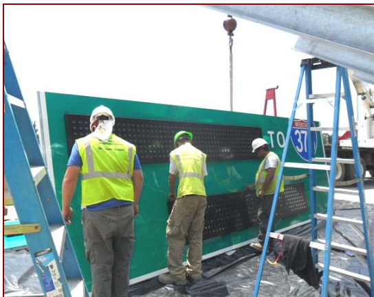
Job No.: 09-19-00, Maryland Department of Transportation @ Navigational Aids at Various Facilities: Foreman Doug Hart and Laborer Riggaberto Granados install white navigational lighting on the Governor Harry W. Nice Memorial Bridge in Charles County, MD.
