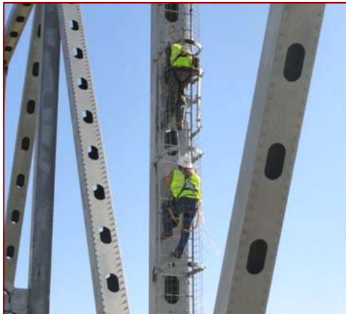
Job No.: 09-19-00, Maryland Department of Transportation @ Navigational Aids at Various Facilities: Foreman Doug Hart and Laborer Riggaberto Granados install white navigational lighting on the Governor Harry W. Nice Memorial Bridge in Charles County, MD.
