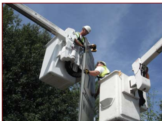
Job No: 10-23-00, South Carolina Department of Transportation @ Spartanburg and Cherokee Cos Signing: Foreman, Fred Garrett and Chris Land installing speed limit signs.
